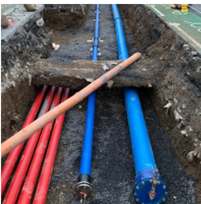
Service ducting for utilities LV/MV ducting, Firemains, Watermains
