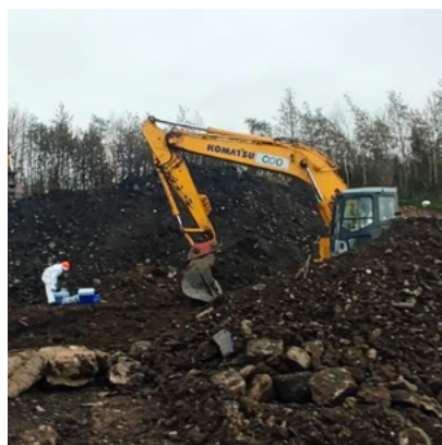
Bulk excavation including management of hazardous waste removal
