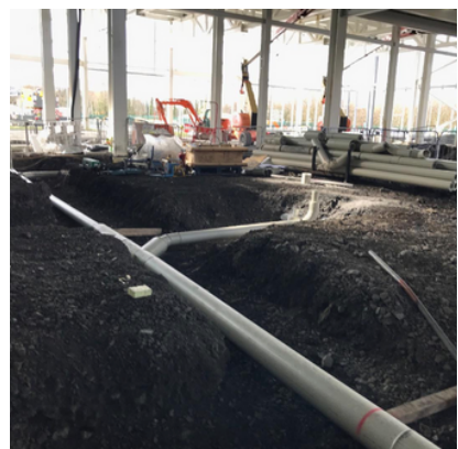
Underground drainage (Foul & Storm)
